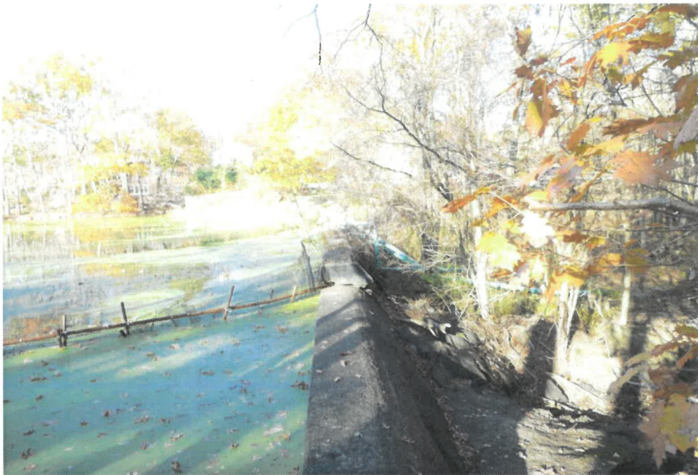
Photo 2 Dam ID# 213-0412 Westchester Lake Dam 11/06/2020 Dam crest and spillway crest
