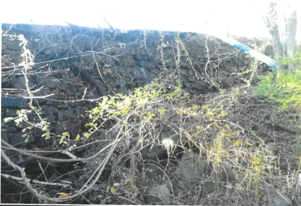
Photo 6 Dam ID# 213-0412 Westchester Lake Dam 11/06/2020 Downstream face of the dam
