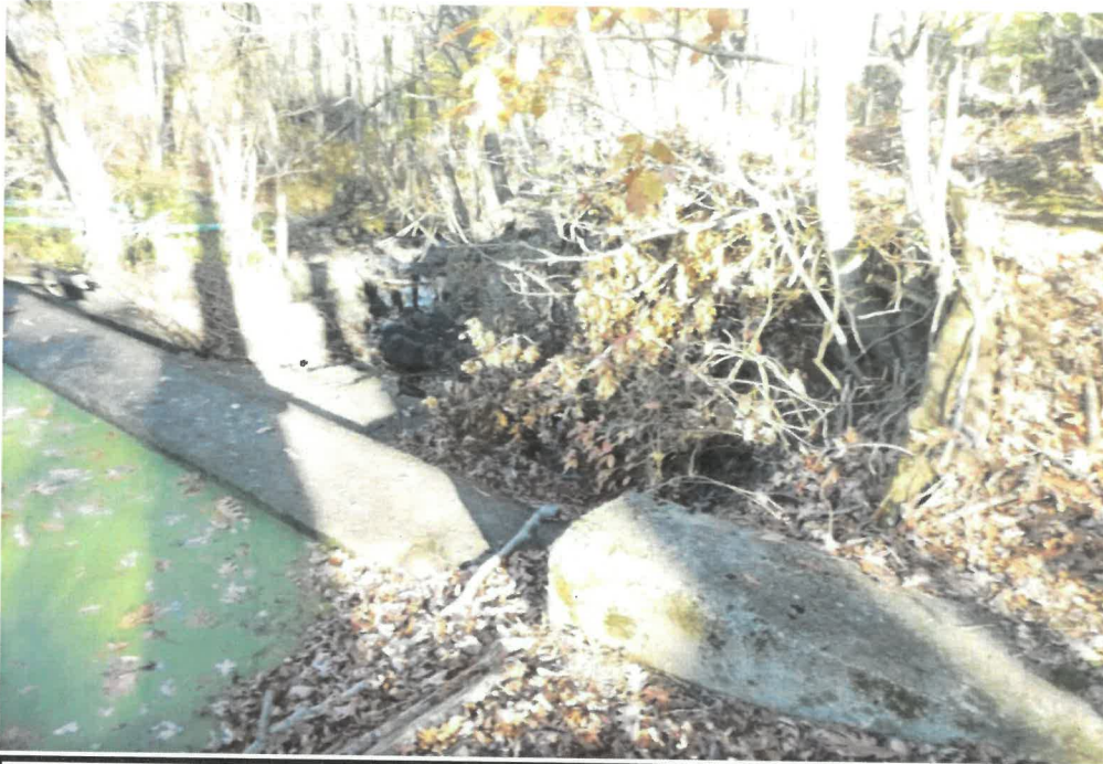
Photo 3 Dam ID# 213-0412 Westchester Lake Dam 11/06/2020 Right side of the spillway
