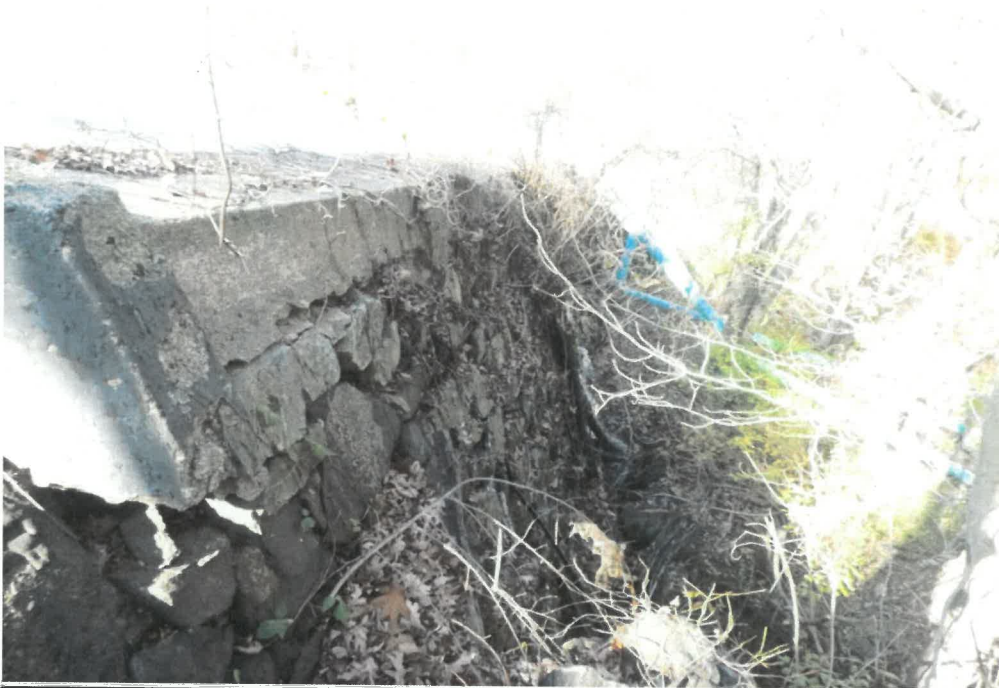
Photo 5 Dam ID# 213-0412 Westchester Lake Dam 11/06/2020 Downstream face of the dam
