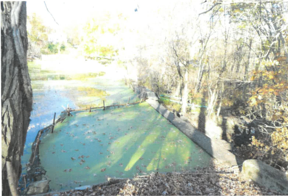
Photo 1 Dam ID# 213-0412 Westchester Lake Dam 11/06/2020 Upstream face of the dam
